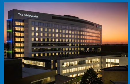
MetroHealth Campus Transformation Cleveland, Ohio
